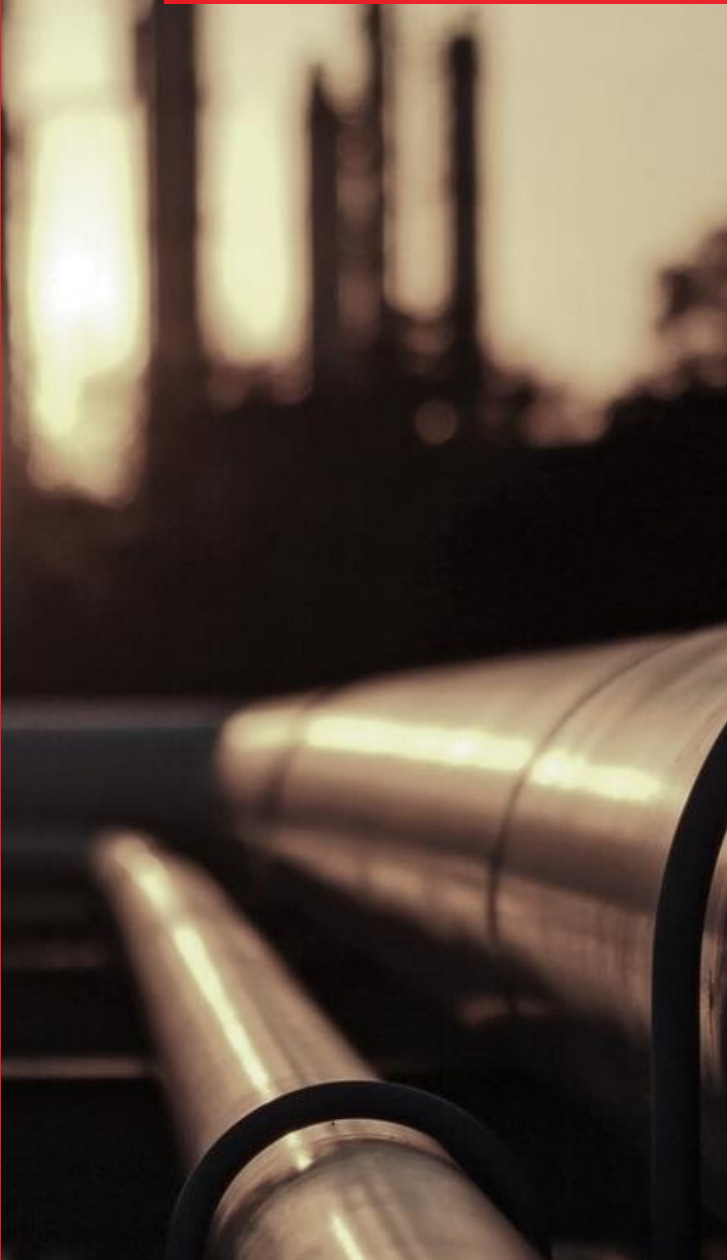
Pipelines, industrial areas (refineries)
